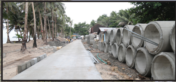
Road Widening in Bulabog, Aklan
